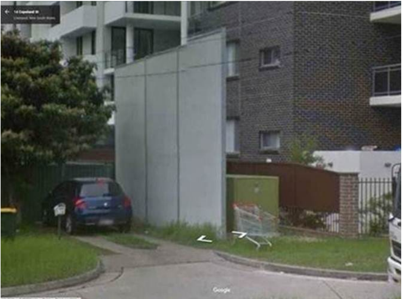
Fire wall constructed for padmount substation at 18 Copeland Street Liverpool. Source: Google Maps Street View.
